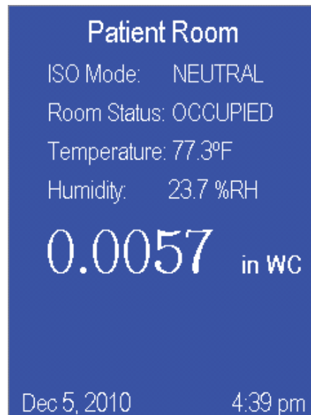
Fig 4. Main display shows isolation mode, room status and differential pressure.
